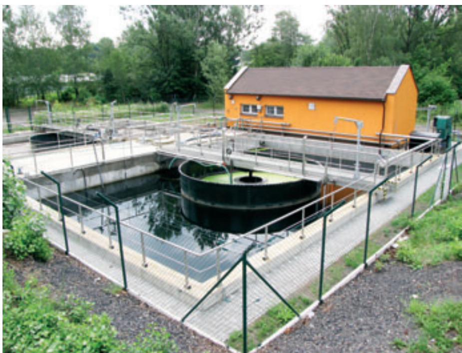
Obr. 6: ČOV Heřmanice II
