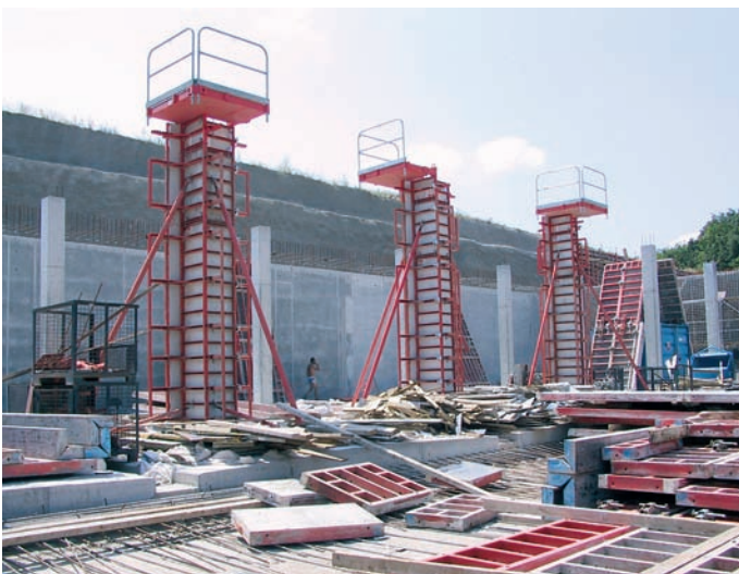
Obr. 6: Betonáž VDJ Lobzy
