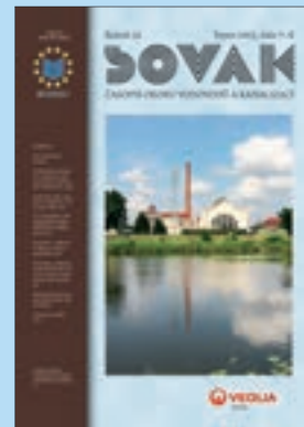
Cover page: The Káraný Waterworks. Operator: Pražské vodovody a kanalizace Company (Prague Water Company)
